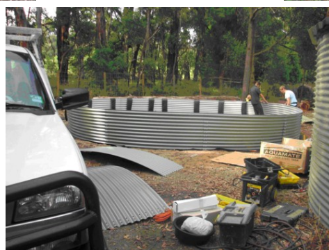
New tank being installed images M.Faram
